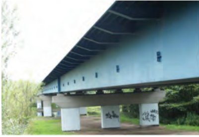
Photo 1. System with zinc rich epoxy primer, epoxy coating, polyurethane coating
