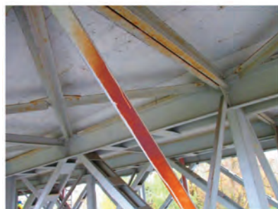
Photo 7. Old-generation thermoplastic system with primer pigmented with minium and chromium compounds
