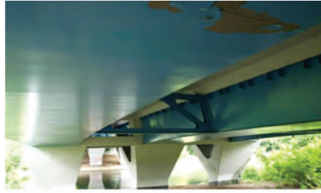
Photo 2. System with zinc phosphate epoxy primer, epoxy coating, polyurethane coating
