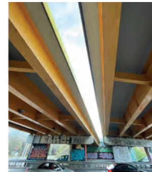
Photo 6. System with zinc ethyl silicate primer, sealer, epoxy coating, polyurethane coating
