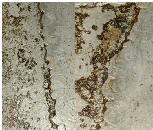
Photo 1. Corrosion pitting on internal surfaces of storage tanks
