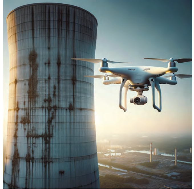
Fig. 2. Scanning the location and type of corrosion damage on a silo shell using a drone
