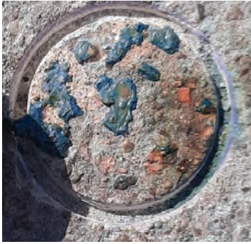
Photo 10. View of a sample detachment during work on a concrete wharf
